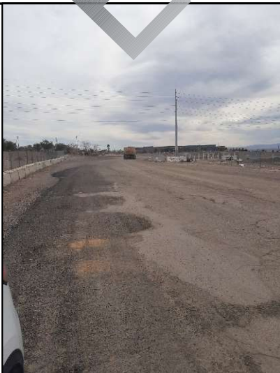
Hollywood Pit 3- Water Truck.jpg
